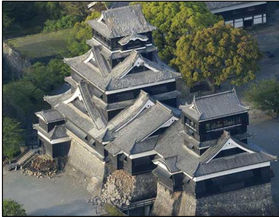
Kumamoto Castle partially destroyed
